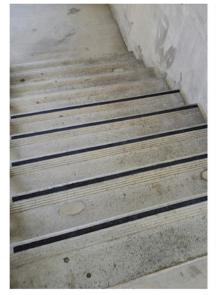
anti-slip coatings to apply. Ideally, the formulation could be applied to a wide range of substrates, resist shrinking and retain aggregate to improve traction and endure many years of wear. Given the large square footage and number of stairs involved in many projects at commercial properties, the time to complete any prep work and apply the coating should be minimized to keep costs down.
