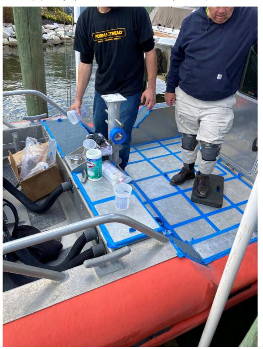
The coating type can be quickly and easily applied without a primer, minimising cost and disruption
